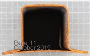
Unpainted omega After corrosion
